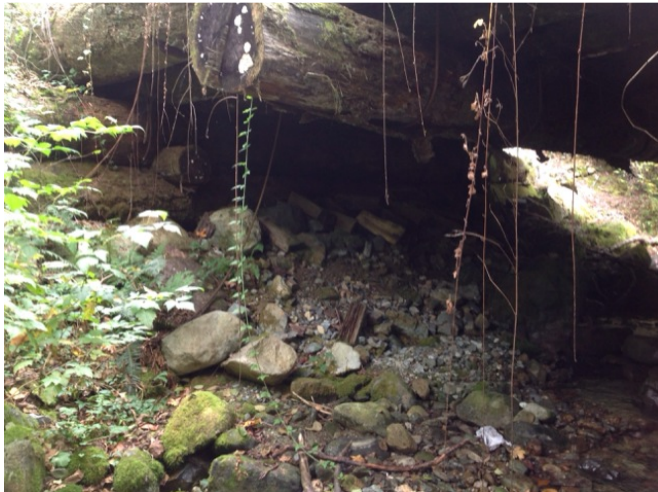
Right Bank Abutment when facing downstream
