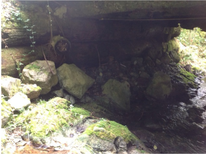
Left Bank Abutment when facing downstream
